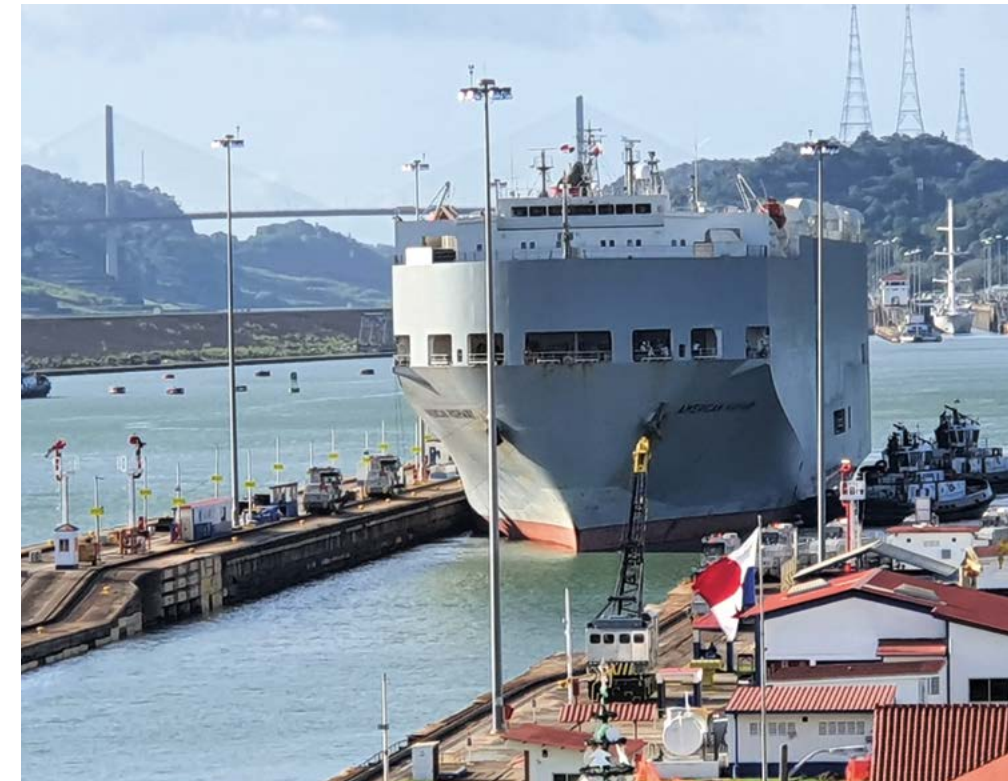
A ship entering the locks of the Panama Canal. The locks act as a massive elevator raising the ships 85 feet above sea level.
